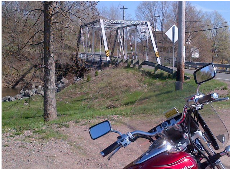
1 lane bridge, Great Village NS
